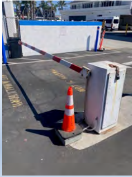
Gate Parking Arm and Housing Replacement
